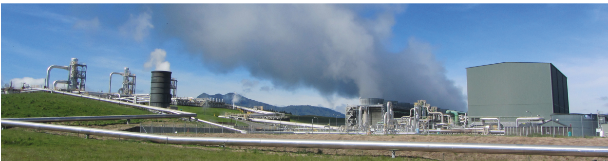
Figure 4: 140 MW e Nga Awa Purua triple flash power station near Taupo, New Zealand.
