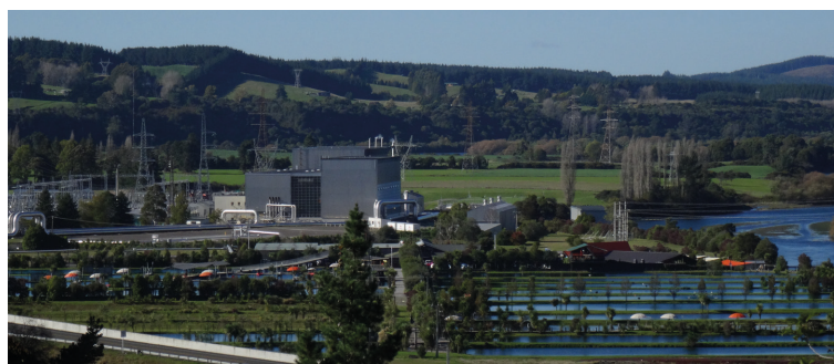
Figure 1: Wairakei geothermal power station and aquaculture
